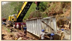
In the meanwhile, the first girder in BFR was brought to the site and was lifted by Crane and kept in position and slowly it was moved to the edge and lowered on the dummy girder with clinical precision. I really appreciated the perfect work done by the bridge organisation without leaving anything to chance.
