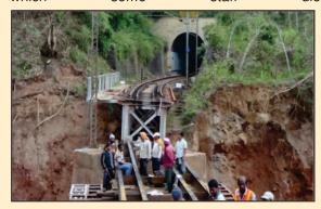
Finally, we reached to the site. There was no connection to the other side of the bridge. It clearly indicated that probably the uprooted trees, slipped heavy rocks and mud had blocked the water passage under the bridge and when the water pressure increased it swept away the track and girder along. The girder, in damaged condition was later spotted three-four KMs away from the site in KR section.
